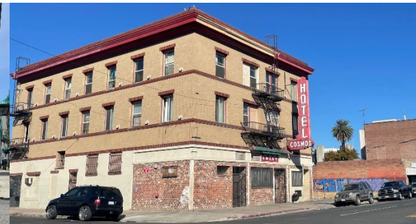
Hotel along San Joaquin Street
